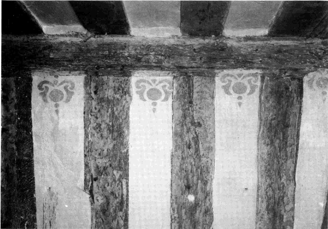
Elms Farm, Mendlesham: ground floor room. Stencilled decoration on north wall.
